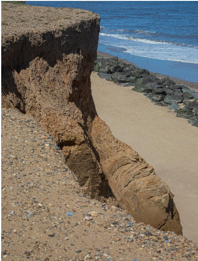
Collapsed edge to beach ramp showing sheer drop to beach
